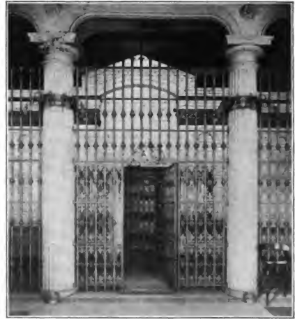
Safe Deposit Vaults.
